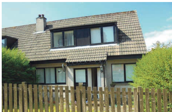
FORMER TARBERT POLICE HOUSE, SCHOOL RD, TARBERT, PA29 6TE OFFERS OVER £90,000
