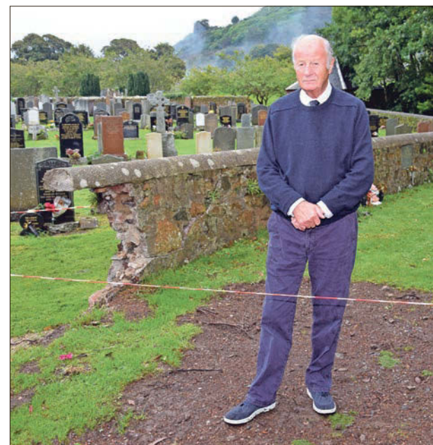
Mr Baxter beside the broken section of wall which is now cordoned off. 50_c38cemeterywall01
