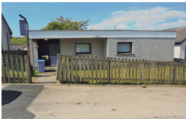
FORMER TARBERT POLICE OFFICE, SCHOOL ROAD, TARBERT, PA29 6TE OFFERS INVITED
