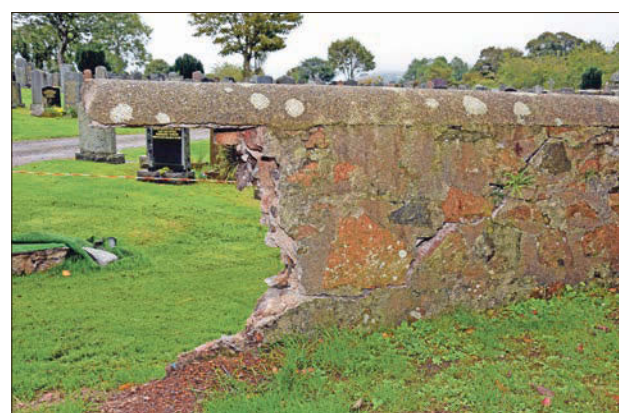
There is a large crack on the remaining section of wall. 50_c38cemeterywall02
