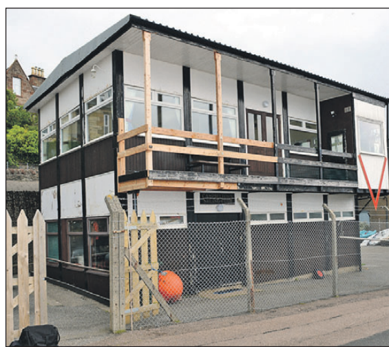
The current Campbeltown Sailing Club building. 25_c25seasports02
