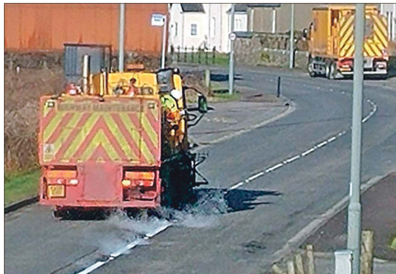
The white lining machine at work in Muasdale.
