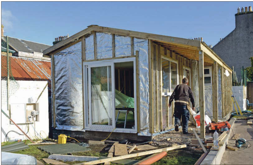
Building works on CLTC's clubhouse.
