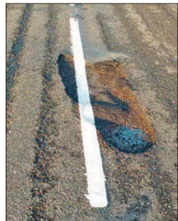
A white line painted across a pothole at Muasdale on Tuesday afternoon.
