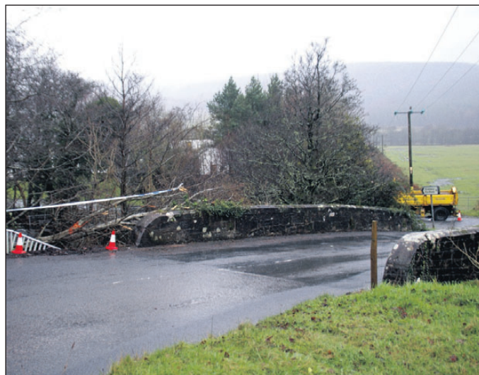
The NAC grit lorry at the Ross Road junction with two burst tyres after being in collision with the Monamore Bridge in the early hours of Sunday morning. 02_b51grt01
