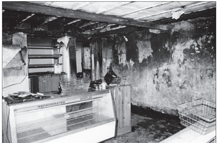
The interior of Pirmill Post Office after the fire. b50twe03
