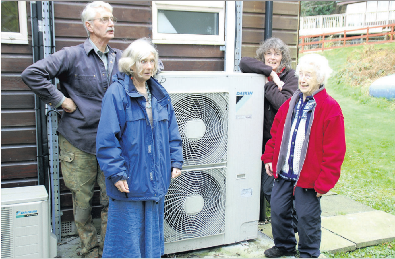
Corrie Hall committee members John and Jan Inglis, Rachael Phillips and Margo Wheeler with the new energy efficient heating system. 01_b46cor01
