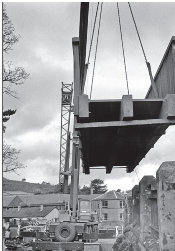
The new pedestrian footpath beside the Arranton bridge in Lamlash was lowered into place on Wednesday. b46twe03
