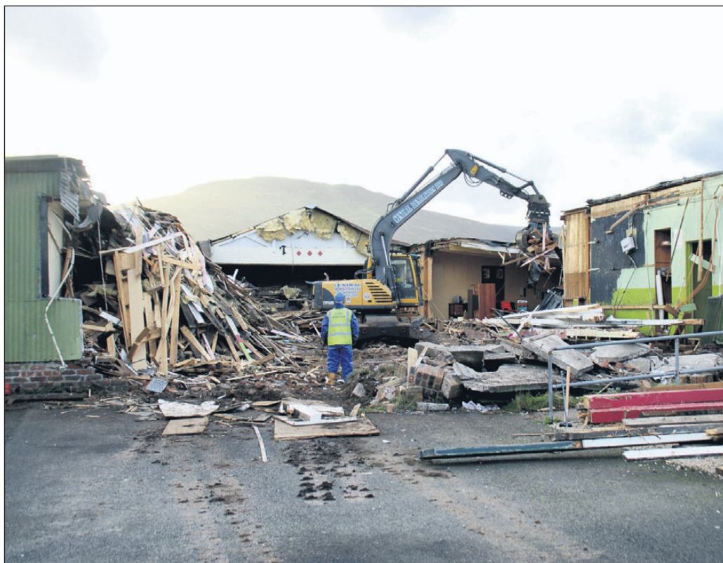
Lamlash Community Centre under demolition this week. 01_b44com01
