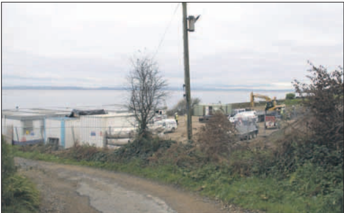
Work progressing at the site of the sewerage treatment plant at the southern end of Whiting Bay village. 02_b44sew01
