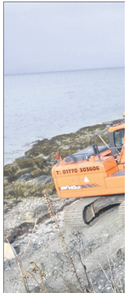
Workmen filling gabion cages on
