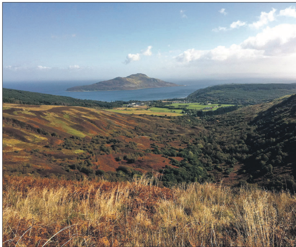
The main intake point for the hydro scheme will be high up Benlister Glen.
