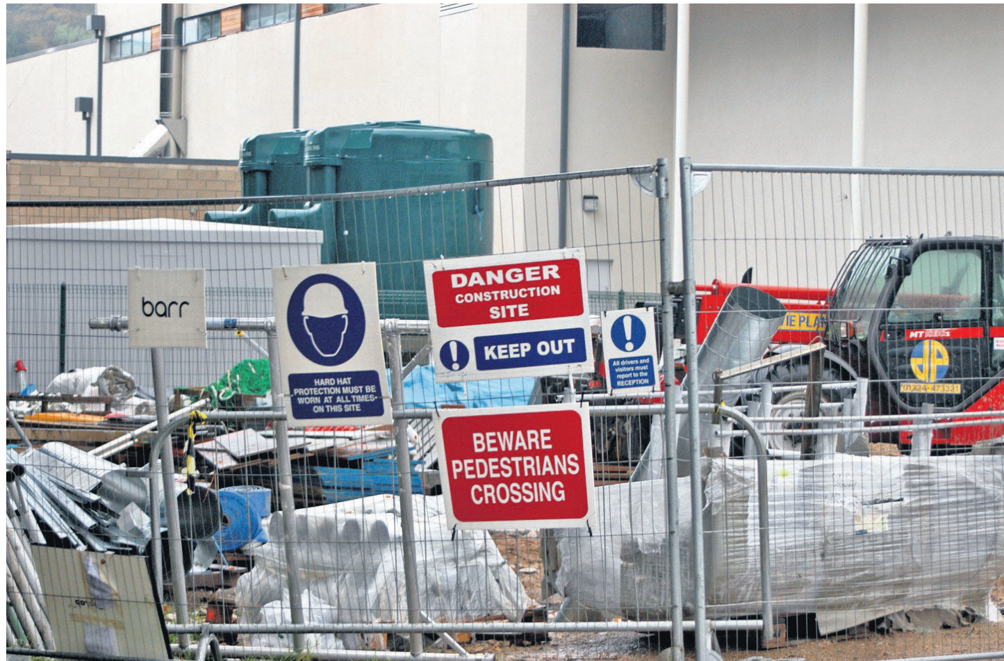
The builder's materials piled up outside the new school this week confirm it is a long way from ready. b40sch1
