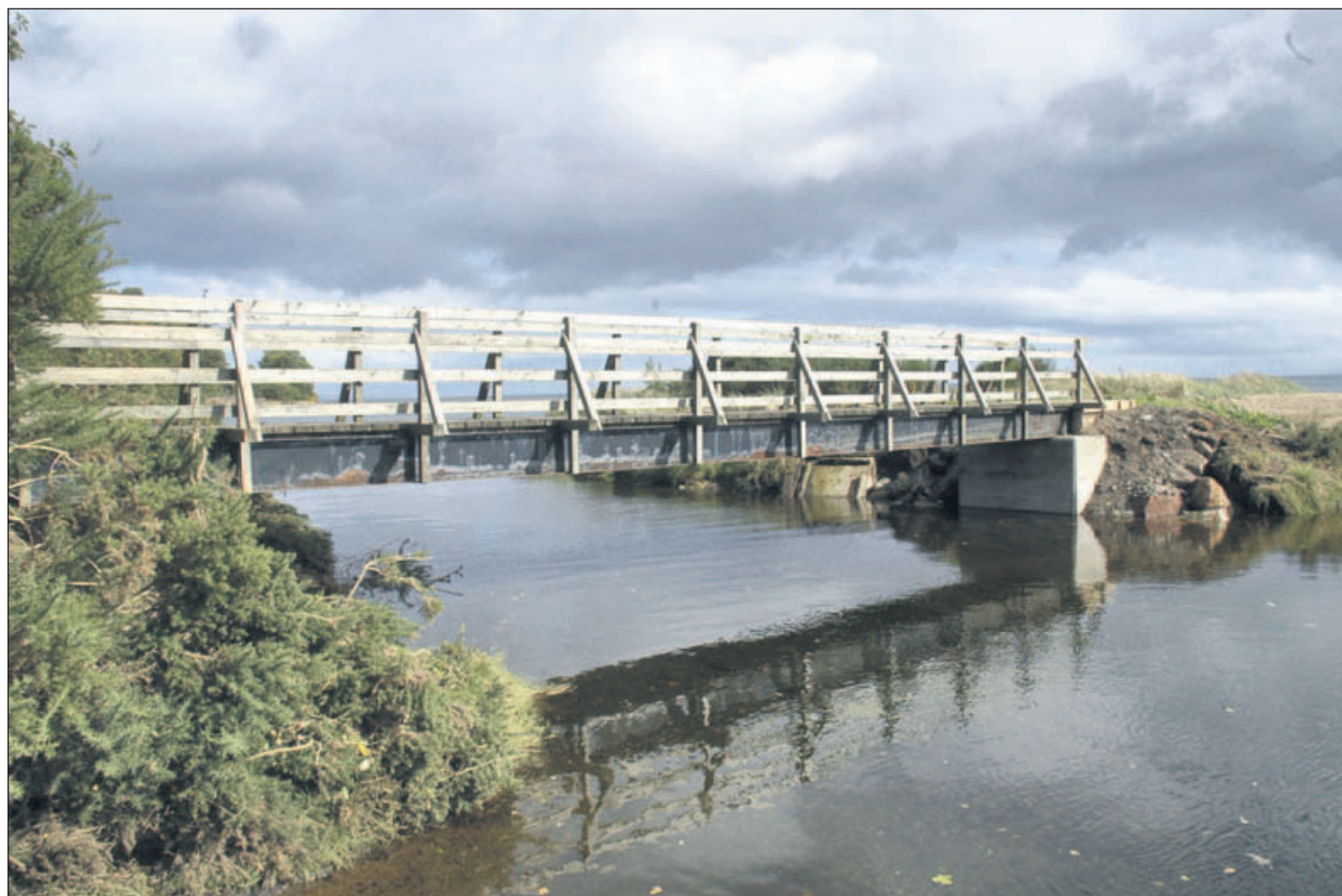
The Cnocan Bridge, re-instated this week. 02_b39fis02
