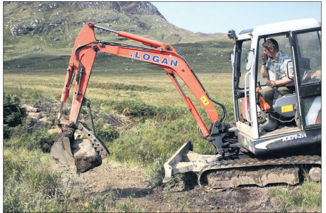
Carrying out repair work using stone from the site. b38ste02
