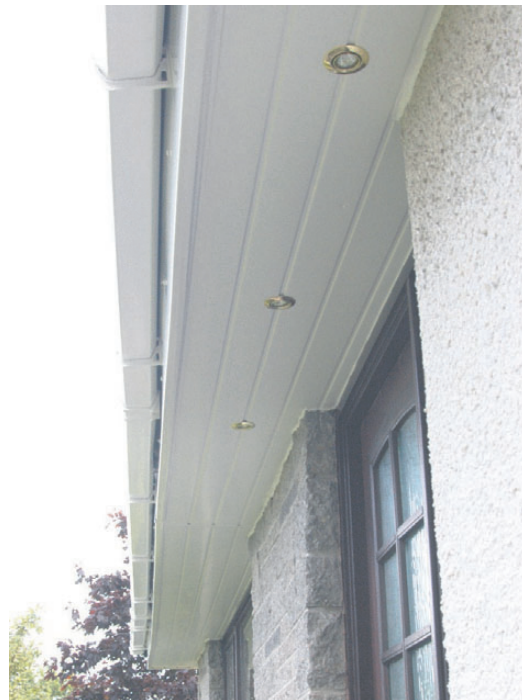
Complete roof lining at Hawksbridge Corrie
