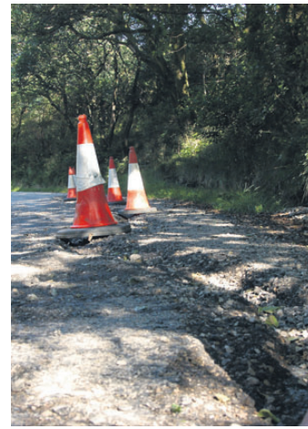
Road damage at Ross Road. b34fl005
