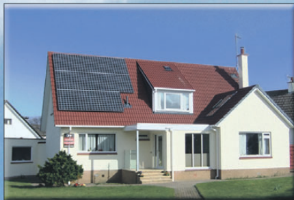
3.9kWp System in Ayrshire
