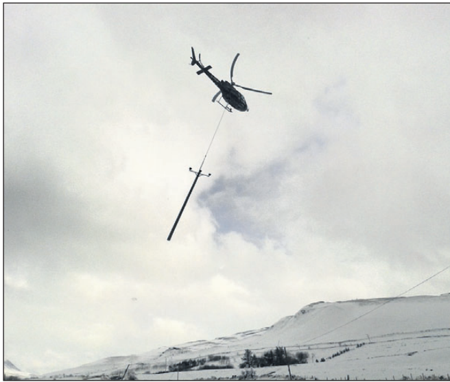
Above: A helicopter airlifts a new pole. Photo SSE
