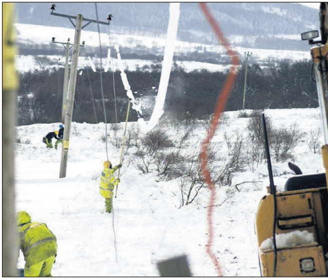
Above: Clearing ice from the power lines. Photo SSE
