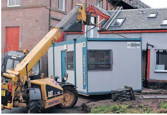
The Arran Youth Foundation cabin being uplifted from Jimmi the Barber's in September before being sited behind Brodick Library. b06cab01
