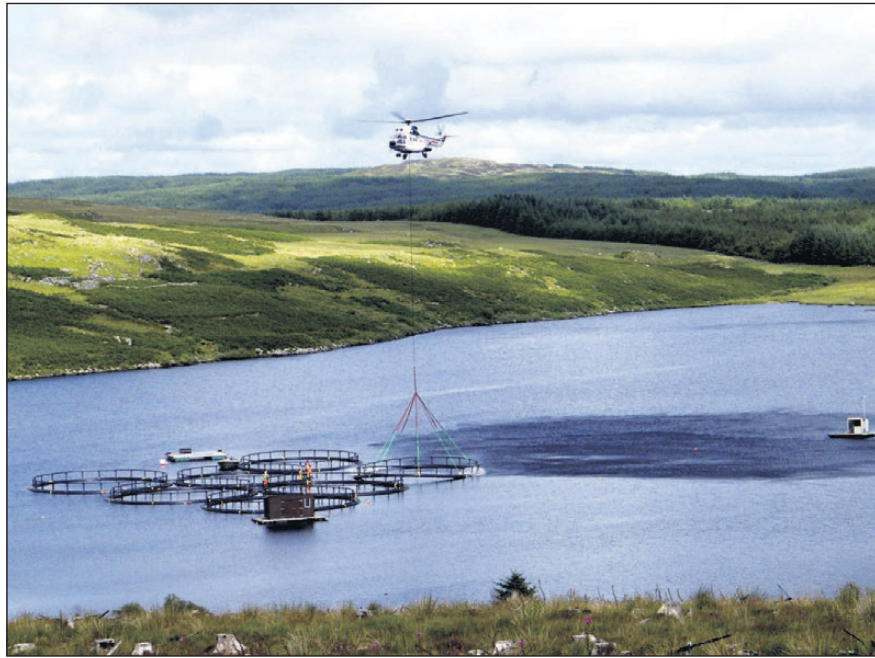
A logistical headache: 2.7 tonnes of salmon pens were flown five miles over North Kintyre by helicopter.
