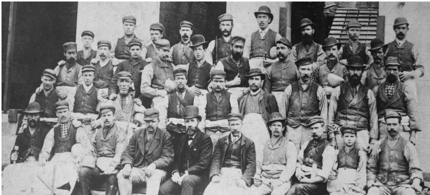
This photo from 1884 was handed in by Don Dennis of Achamore House, Gigha. It shows the team of workmen employed by Jackson Brown & Co of Glasgow to build Achamore House.
