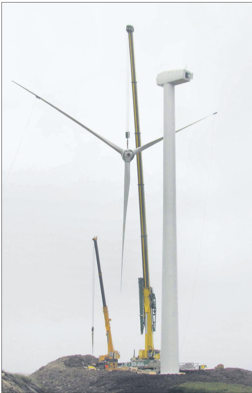
The first wind turbine was installed at Allt Dearg on Monday.
