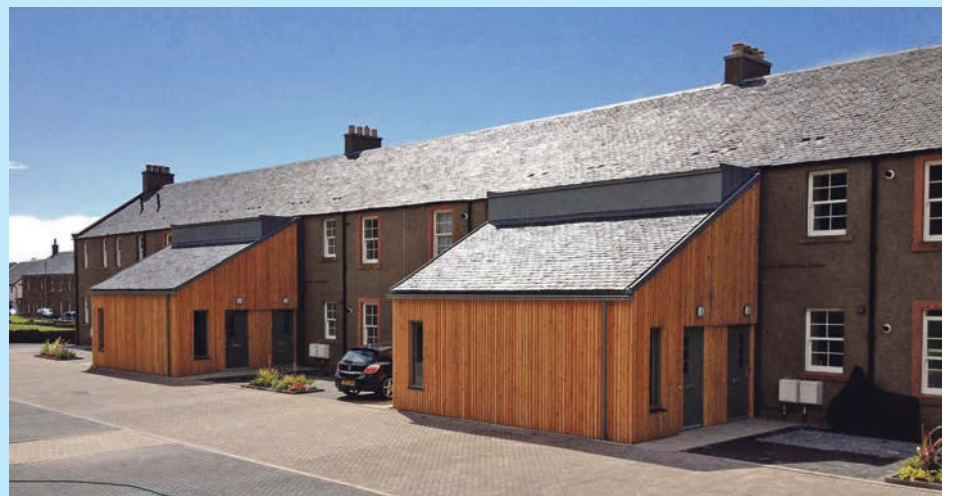
Roofing and slating
