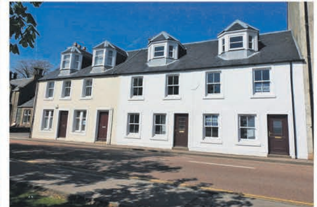
External building painting & renovation
