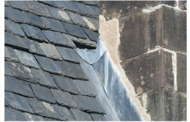
Roof leadwork replacement
