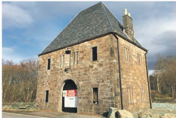
Slate roof renovation - Clock Lodge
