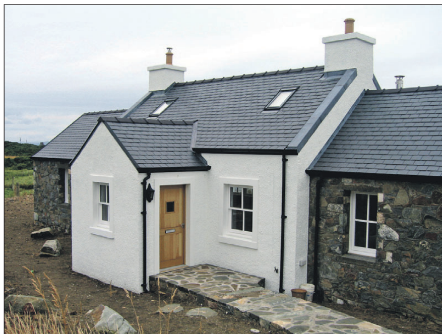
This is a new build kit house built in Sloan's workshop from architects drawings, stone faced and rough cast finished
