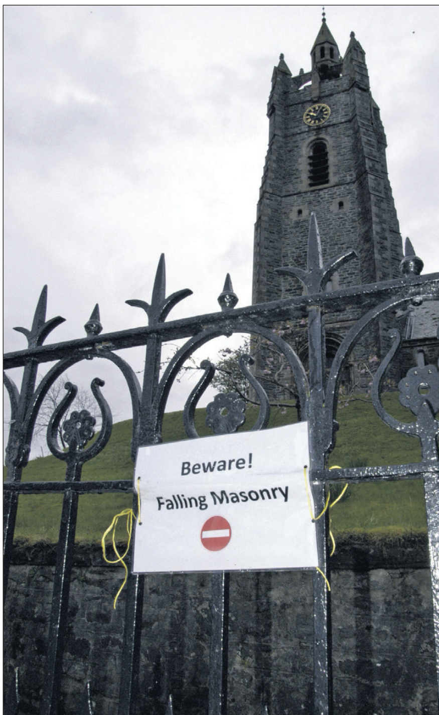
Tarbert Parish Church is going to cost around half a million pounds to repair - at least. 12_a15church01
