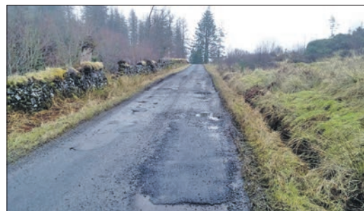
This photo of the B8000 Kilfinan road was sent by Otter Ferry resident Madelon Halley, who said: ‘Locals know where potholes are. It’s going to be a problem once tourists start coming.’
