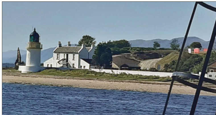
The new bellmouth can clearly be seen to the rear of the lighthouse as viewed from the ferry.
