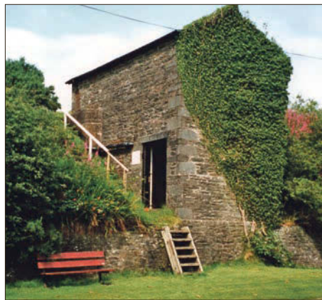
Water waster building, Ardrishaig, in 1996. Photograph: Alison Smedley.
