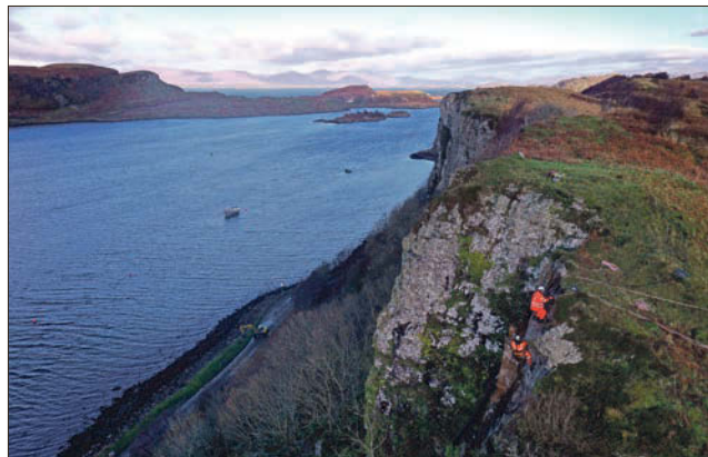
Geo-Rope specialists at work above Gallanach Road.
