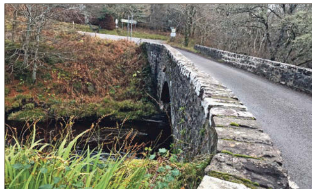
Kilninver bridge has bulges appearing and stones missing.
