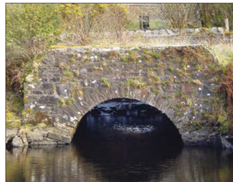
Water supply entering the canal via a culvert at Cairnbaan; and right, a sign indicating a telegraph cable under the canal, near Ardrishaig, Crinan Canal. Photographs: Alison Smedley.
