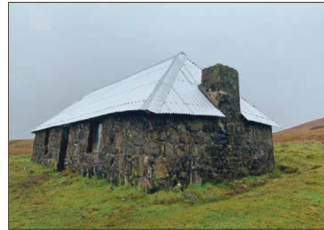
Ollisdal with its new roof in place.
