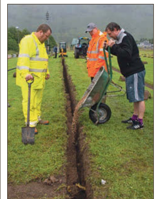
Members of the Fort William FC Committee getting stuck in to drainage works at Claggan Park in July 2020.
