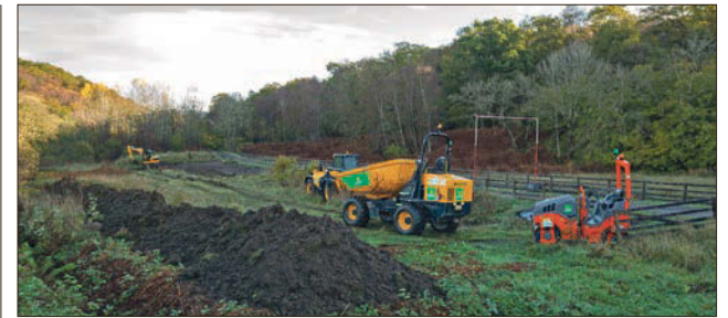
Work has started on the A82 repairs at Kiachnish Bridge.
