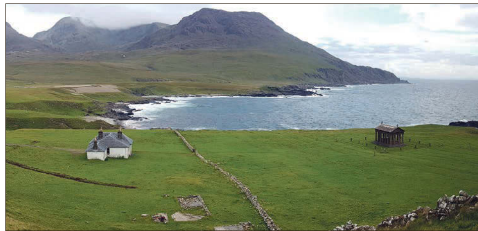
Harris Lodge was built as a sporting lodge in the late 1800s.
