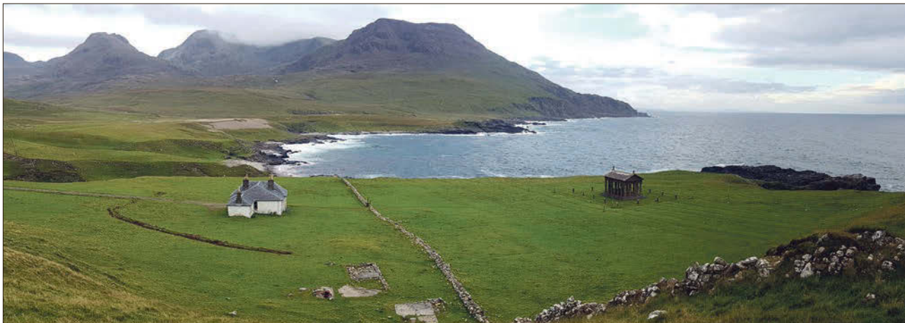
Harris Lodge was built as a sporting lodge in the late 1800s.
