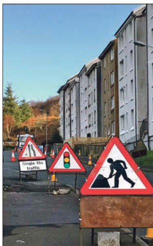
Roadworks in Soroba for pipework improvements by Scottish Water as part of the new water mains project.
