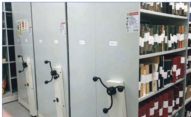
The centre's strongroom. Photographs: Lochaber Archive Centre.
