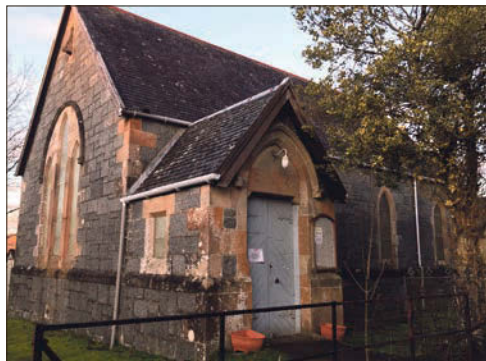
Connel Church Hall sits in the centre of the popular village.
