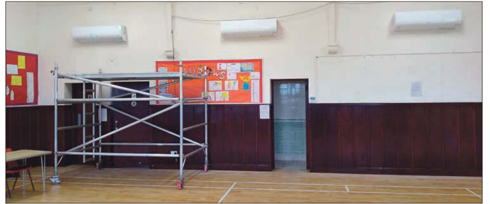
The new energy efficient heaters have replaced the old ceramic wall heaters.
