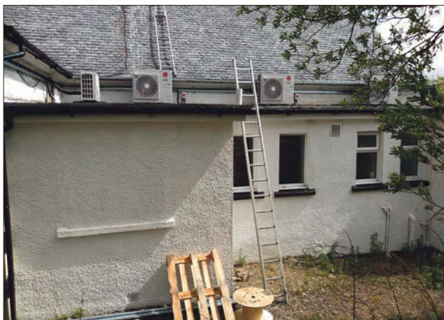
Air source heat pumps are expected to reduce heating costs as well as being more efficient.
