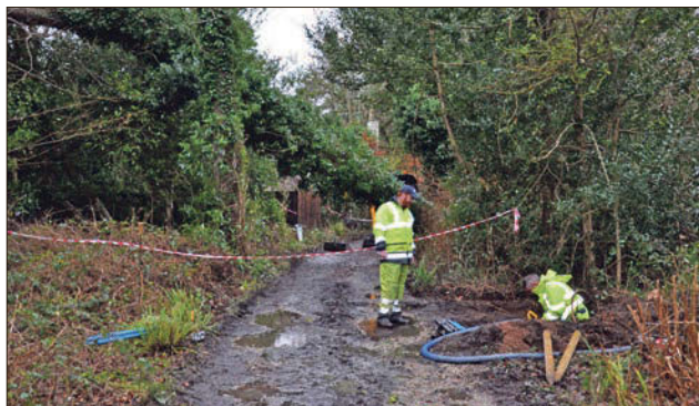
Scottish Water workers investigate a broken water pipe while the fallen tree can be seen behind them. 01_B05corrie02
