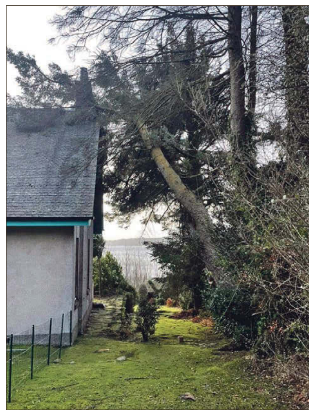
A Lamlash resident had a narrow escape when a tree toppled and leaned against his roof. Photograph: D Steel.
