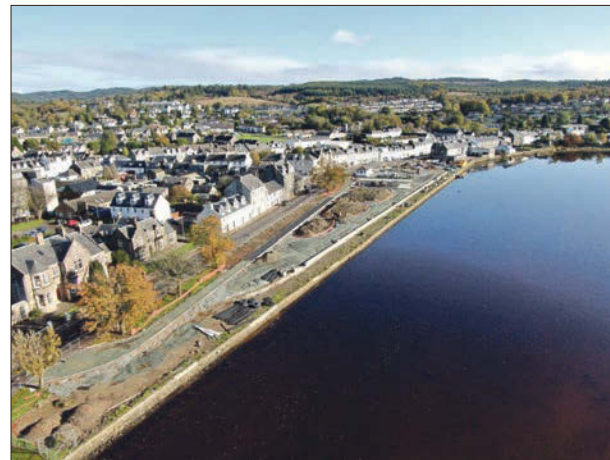
An aerial shot showing the retaining wall parallel to the existing sea wall for a new raised, well-drained ground level along with a new cycle/footpath.
