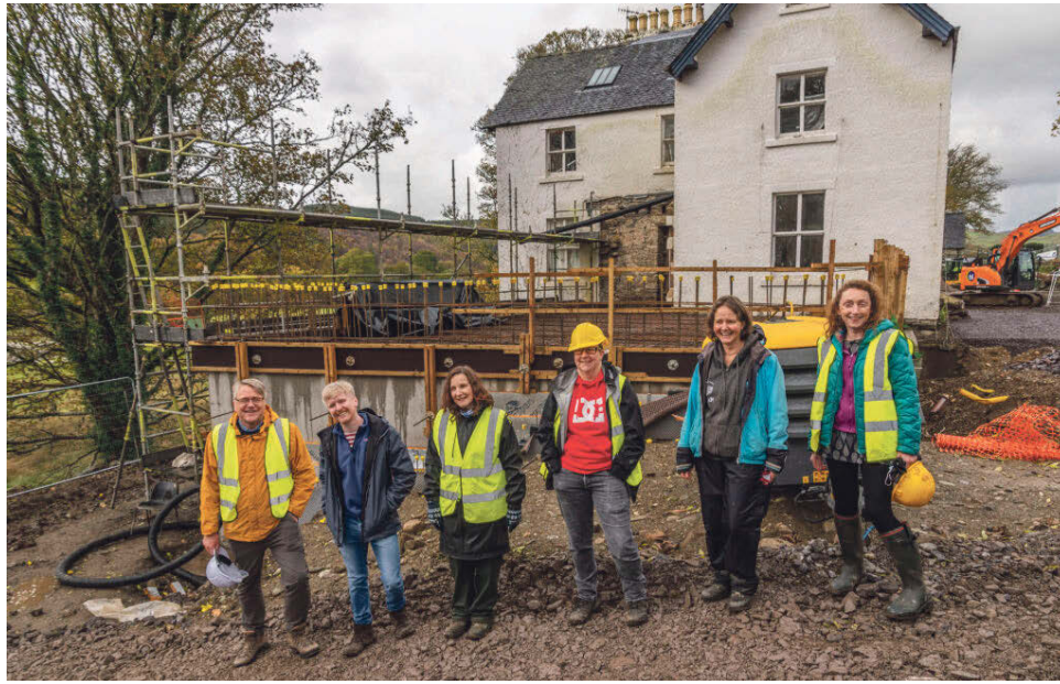
Kilmartin Museum director and curator Dr Sharon Webb MBE, far right, accompanies staff as they visit the construction site.
