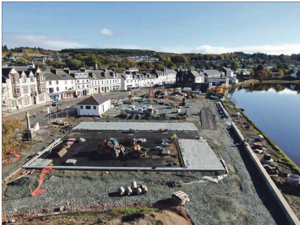
Achnaba stone, quarried locally by MacLeod Construction Ltd, being laid to form an impressive new public space for the town.
