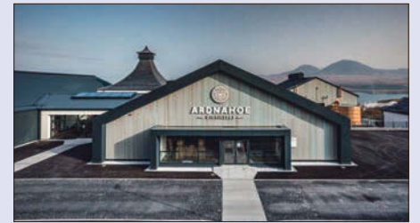
Nine new warehouses are planned at Ardnahoe’s distillery in Port Askaig.
