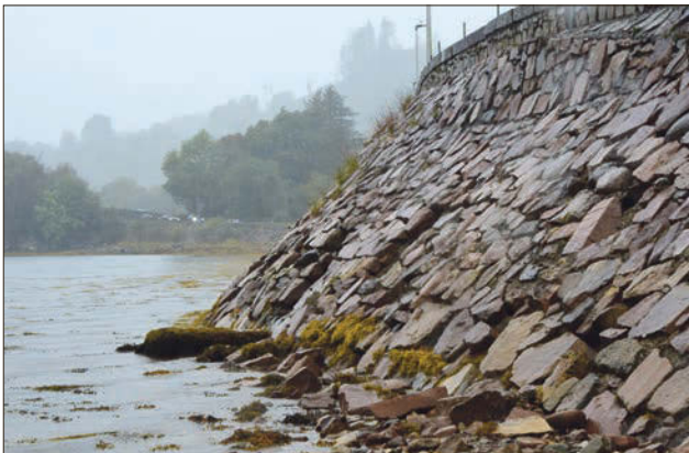
Stones have been dislodged in Loch Fyne storms and the sea wall should be repaired later this year. 51_a42InveraraySeaWall03
