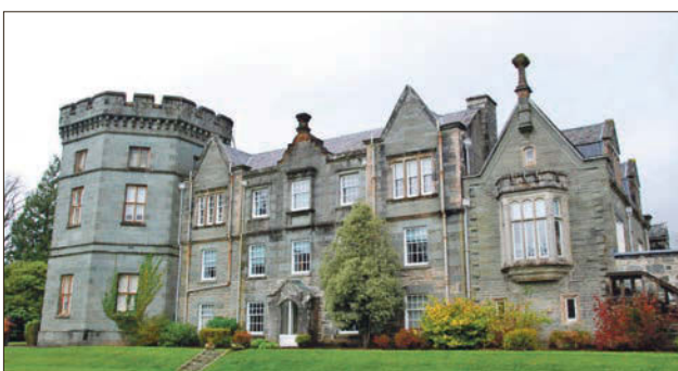
Argyll and Bute Council headquarters, Kilmory Castle.
