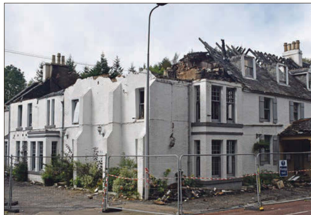
The fire destroyed a large part of the Taynuilt Inn.
