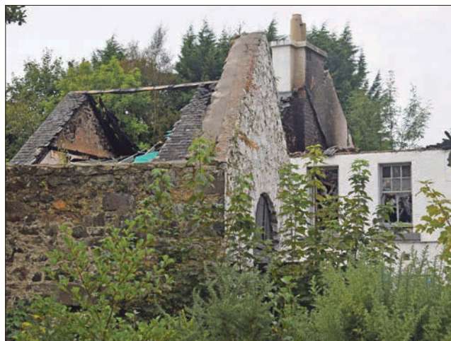
The back wing of the Taynuilt Inn is virtually a shell following last week's fire.
