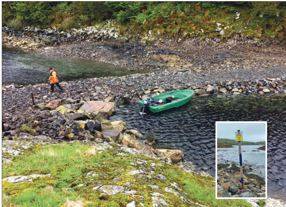
Left: The raised causeway, still above the water level at half-tide. Inset: A sign warning water-users to 'proceed with caution'.
