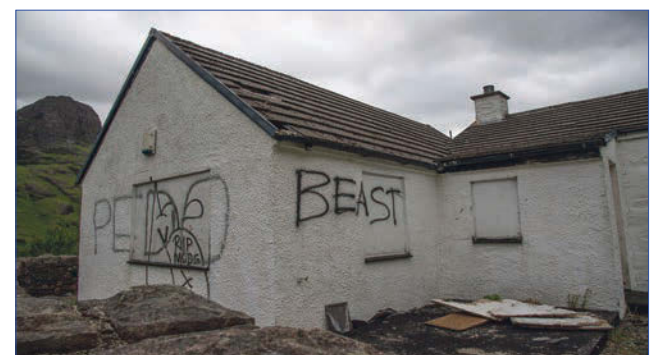
Vandals defaced the derelict house in 2019.
