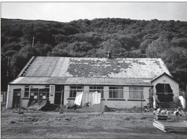
The old Lochranza Hall finally came down this week. Having been stripped the previous week the bulldozers moved in, leaving an open space behind the new hall which was opened last Easter. 01_B38ABTYA02
