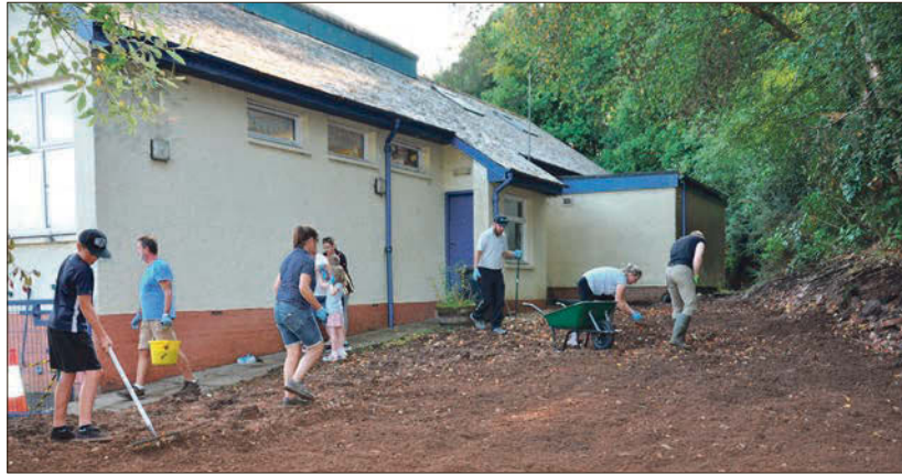
Volunteers rake and unearth stones which other volunteers cart away in wheelbarrows until the outdoor area nears the stage where grass seed can be sown. 01_B35BPS01
