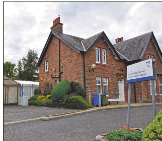
The temporary unit is sited at Brodick Health Centre.
