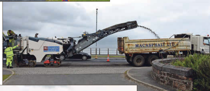
Above: Asphalt is removed from the road and deposited into awaiting lorries. 01_B25roadworks01 Left: Motorists queue at temporary traffic lights, blocking off parking spots and entrances to businesses. 01_B25roadworks04
