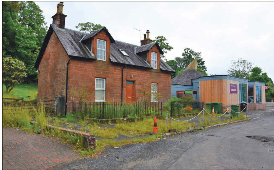
The Pier House and iCentre which would be demolished to make way for the office block.
