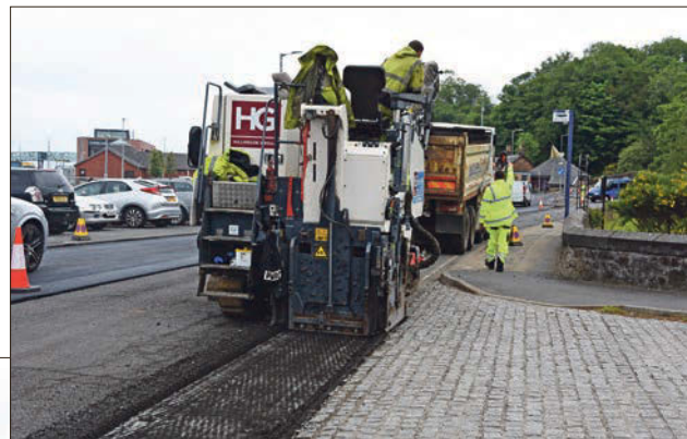
Above: Heavy machinery grinds away the road surface which is then renewed. 01_B25roadworks03 Left: It was one-way traffic while workers resurfaced the road. 01_B25roadworks02
