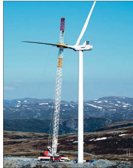
Up to 26 wind turbines proposed for site near Dunadd.
