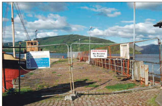
The pier has been closed off to the public for many years as it fell into disrepair. 06_a21InverarayPier04
