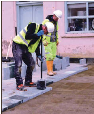
Lochgilphead front green will have stone paving to complement the Achnaba slabs seen here being laid in Colchester Square earlier this year. 51_a11ColchesterSquare07
