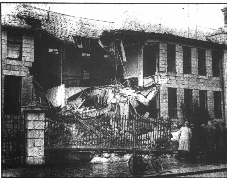
JULY 20, 1940... bomb-damaged Peterhead Academy
